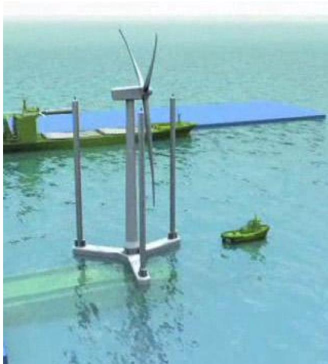
As the platform arrives at its permanent location, preparations are made to begin the jacking up mode. Wedges are removed from the leg guides, the jacking system is rechecked, ballast tanks and pumps are prepared to take sea water and temporary protection and securing devices are removed.
