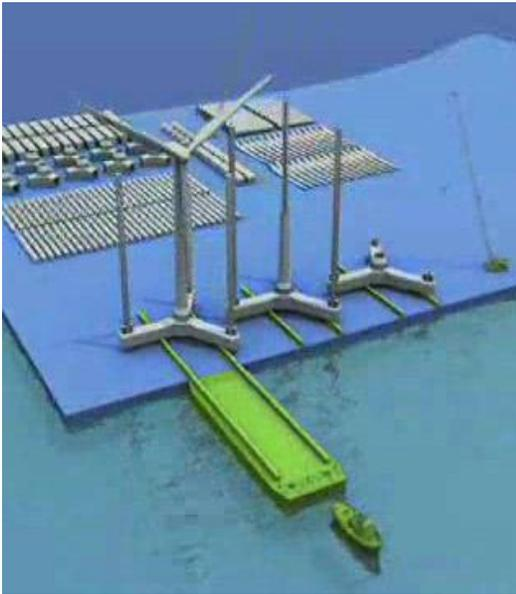
Wind turbines up to 10 MW can be accommodated in the current Titan design. The turbine is assembled on the hull and fully erected before the system is floated. Thus, all construction is performed using land-based lifting equipment.
